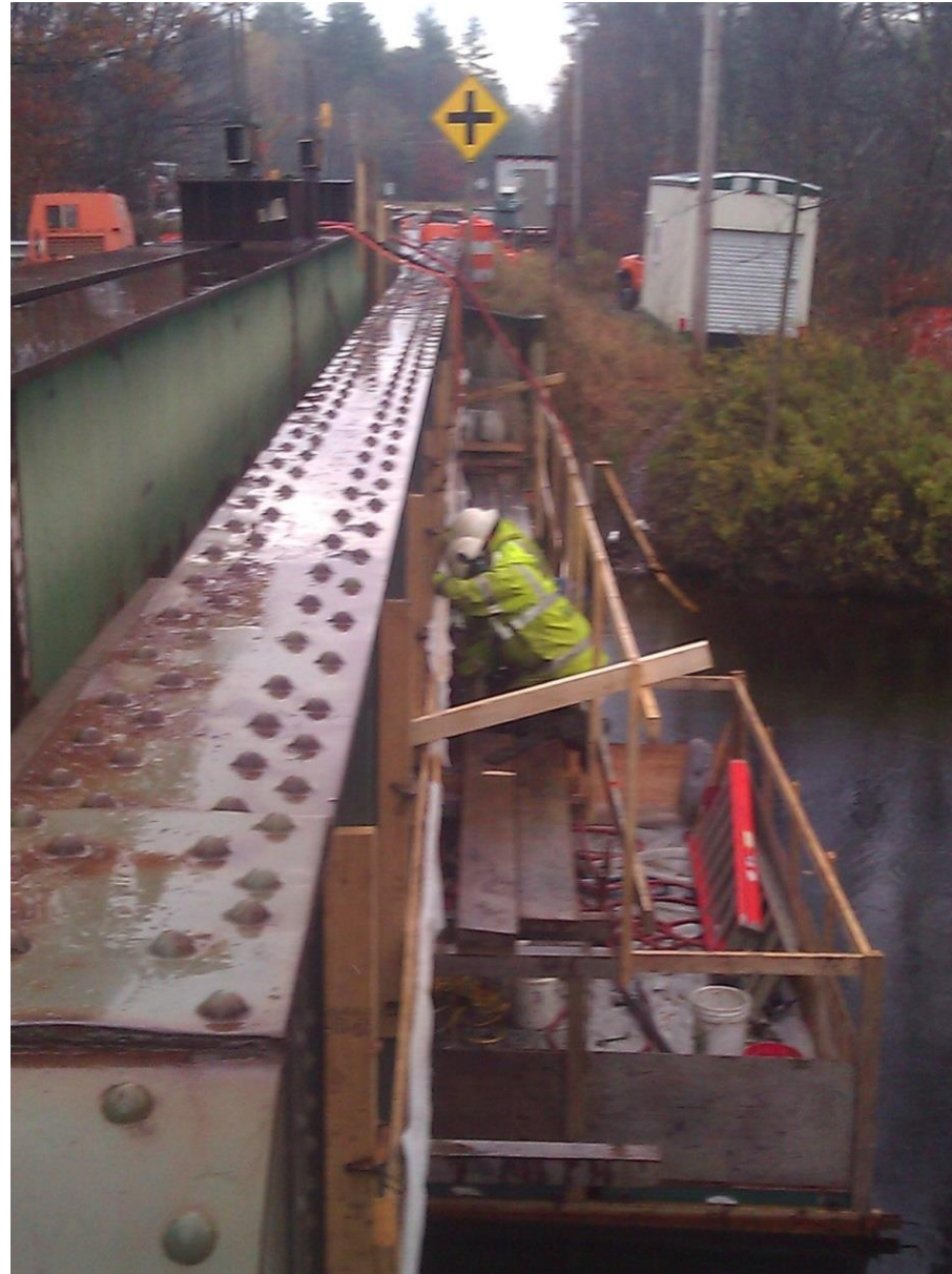
Drilling holes
