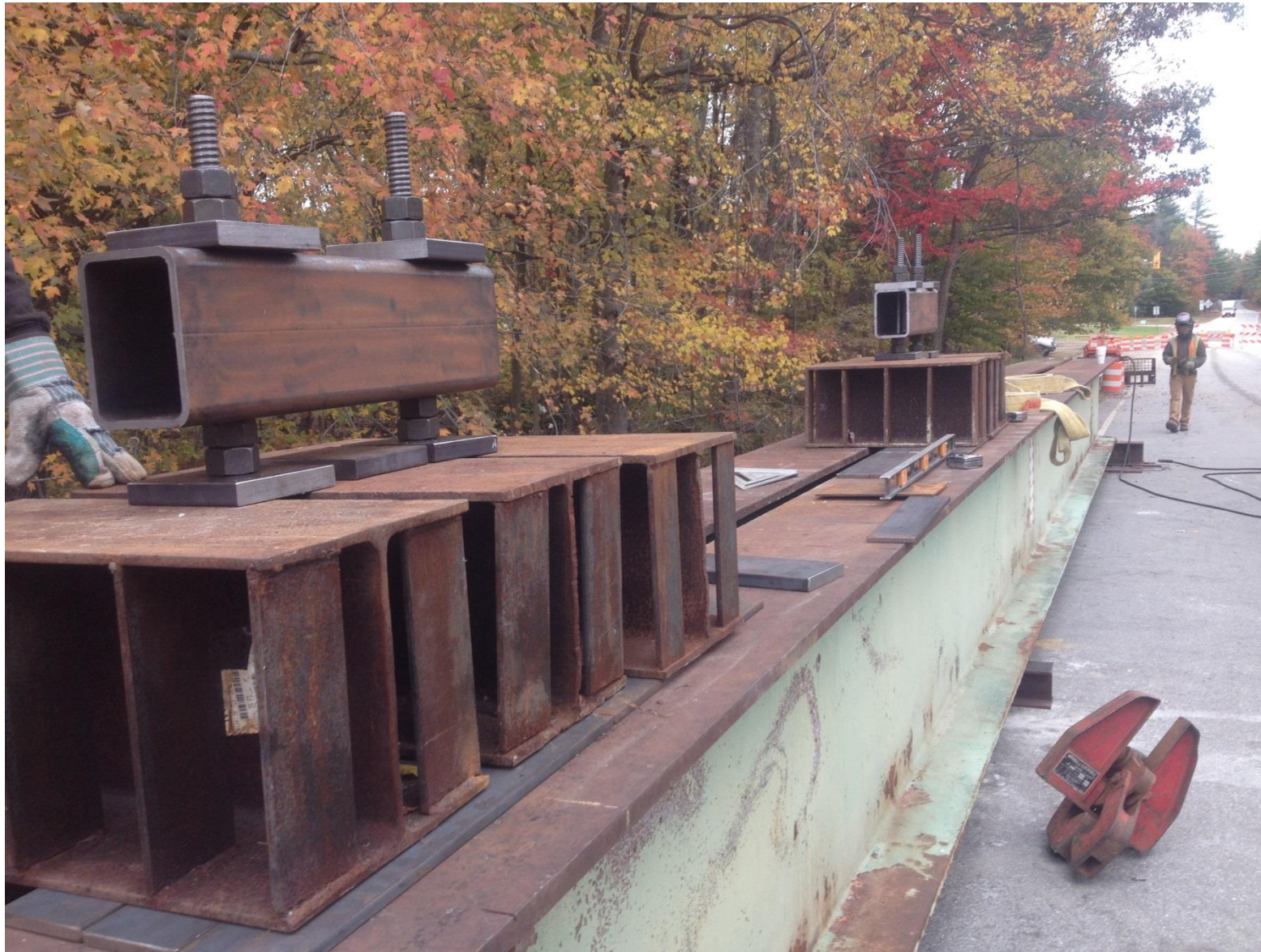
Jacking apparatus in place
