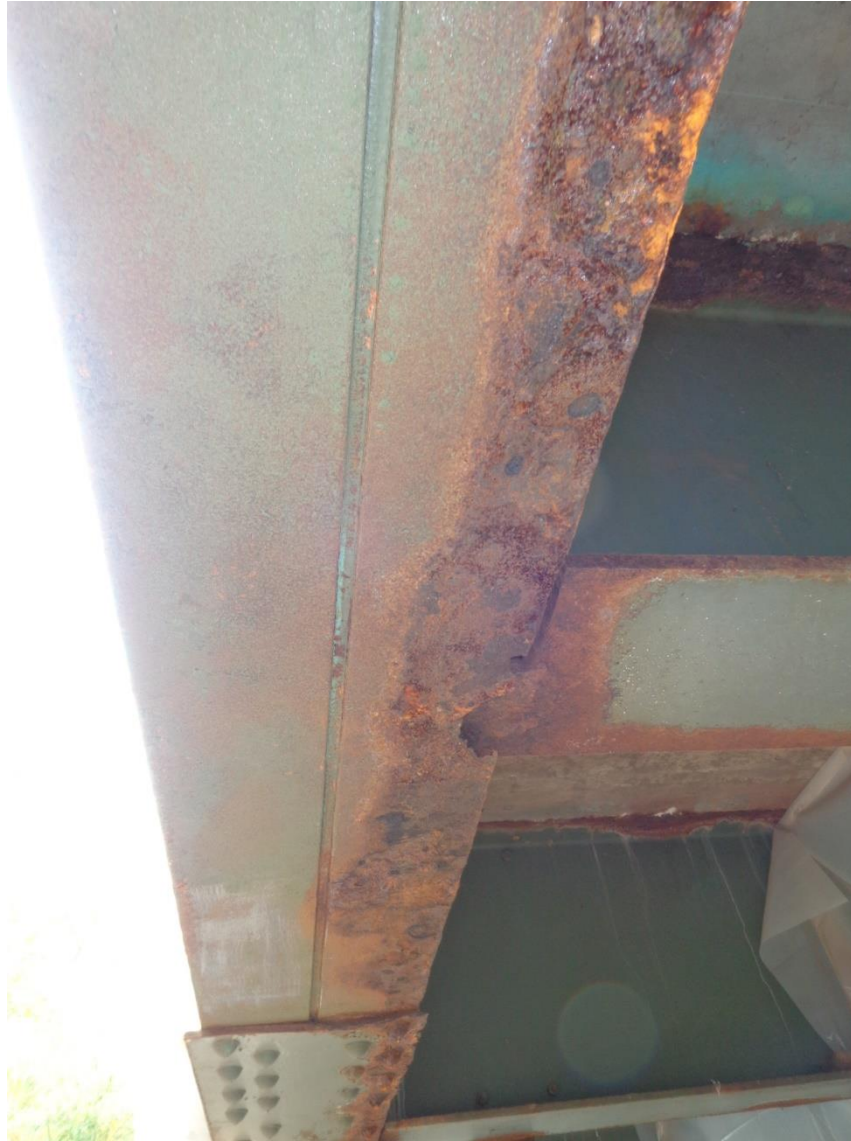
Lower flange section loss in critical area
