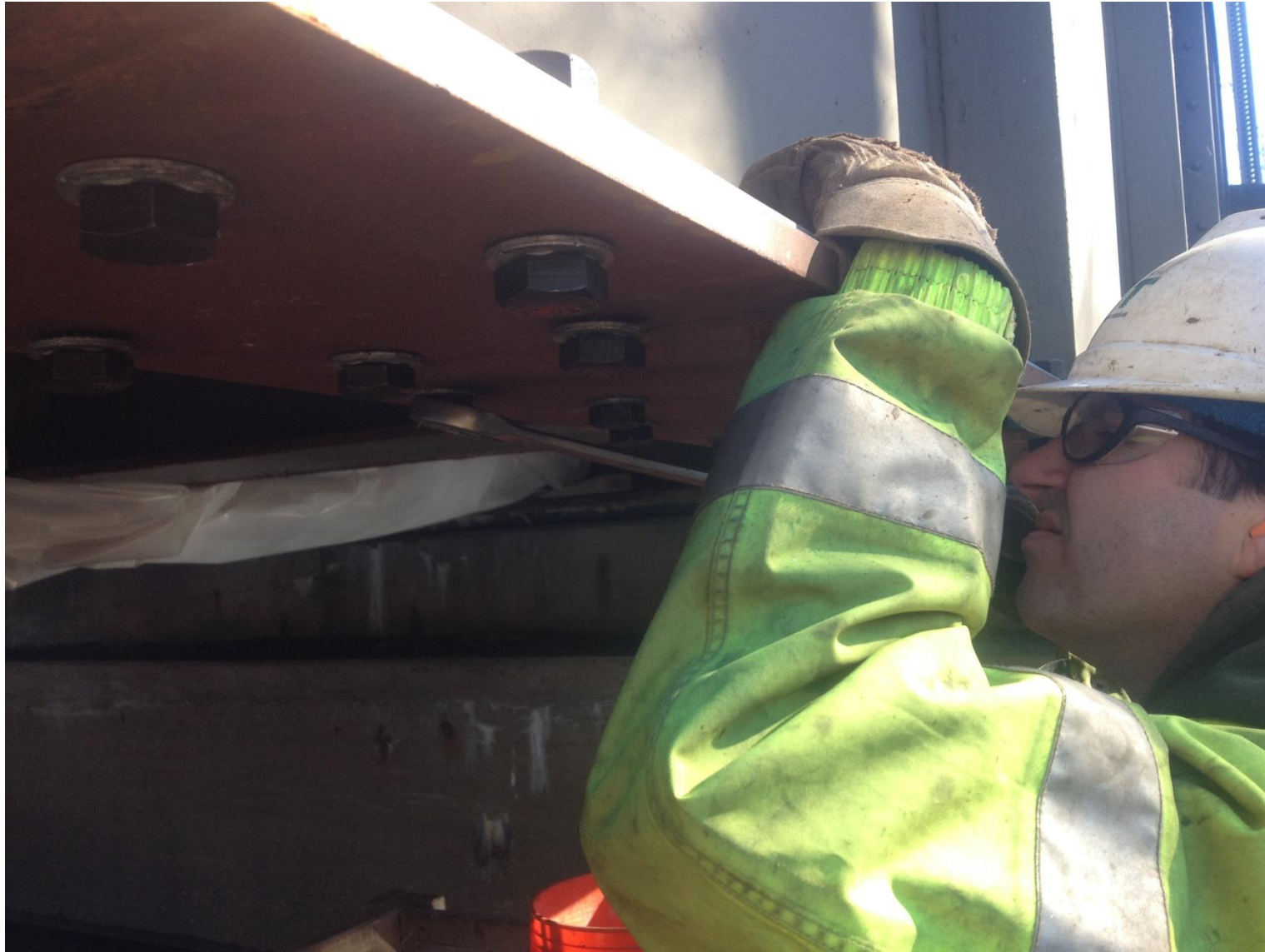
Tensioning bolts
