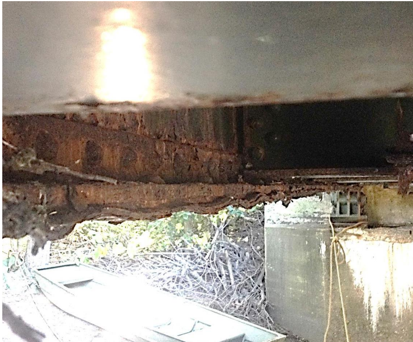
Typical condition of existing cover plate
