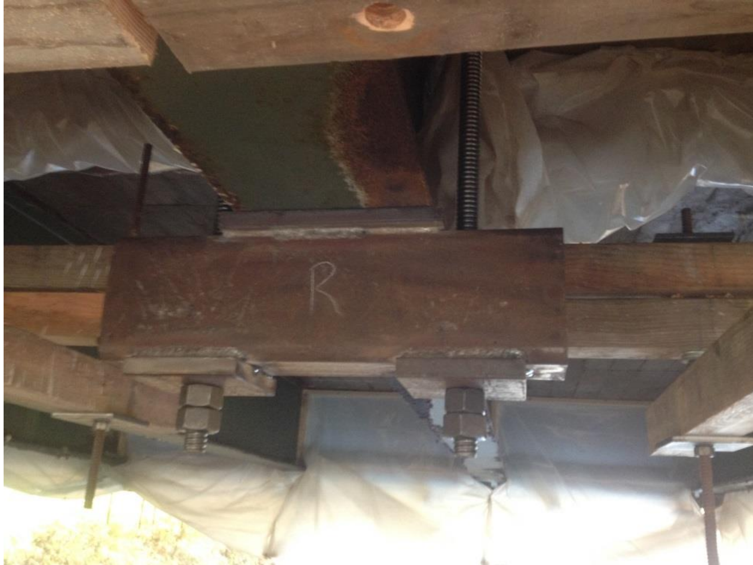
Jacking system at floorbeam
