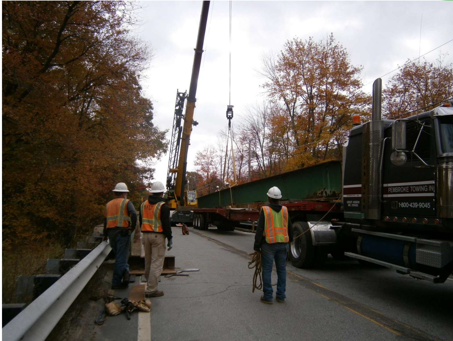
Placing support girders
